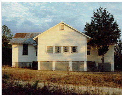
The Shiloh-Rosenwald School before restoration
