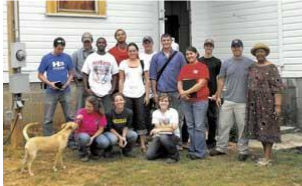
Students of the Design Build Masters Program at Auburn University have been working with SCRF President Liz Sims, far right, to renovate the Shiloh Rosenwald School in Notasulga.
